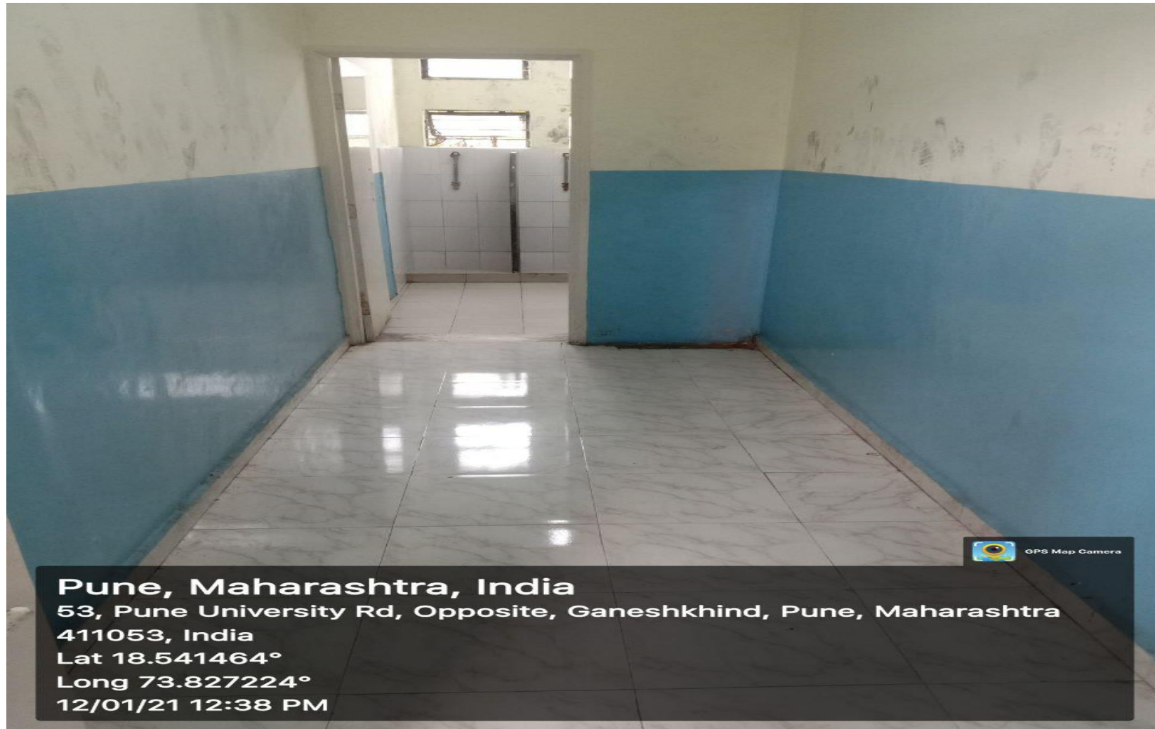
16. Boys Wash Room
